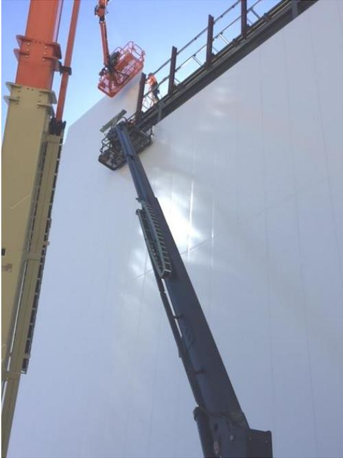
AWIP personnel were on the site to ensure that two custom-designed stack joints on the warehouse were fitted to allow panels to sit smoothly up the entire building. No trim or flashing breaks the exterior plane.
