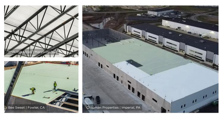
OneDek<sup>®</sup> by All Weather Insulated Panels is an innovative alternative to a traditional multi-layer low slope roof assembly. Replacing steel deck and multiple layers of ISO board insulation, a OneDek assembly requires fewer components and less steps to install, saving construction time, and labor, while providing exceptional energy efficiency for your roof assembly. An industry exclusive 20-year, top-to-bottom full assembly warranty is available.
