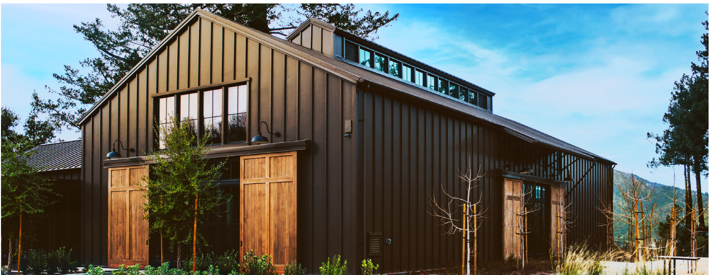
1.5" BATTEN JOINT & MID-PANEL PLACEMENT
